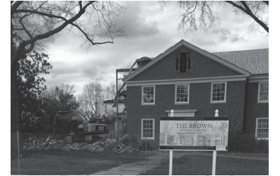
Eggleston's destruction has begun. Photo Credit: Jonathan Walkey
